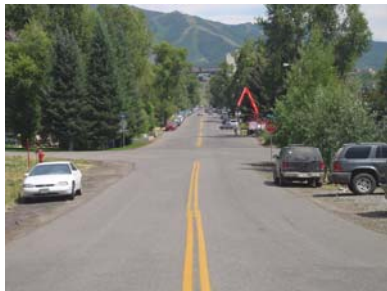
Collector Roadway Example: Oak at 8 th
